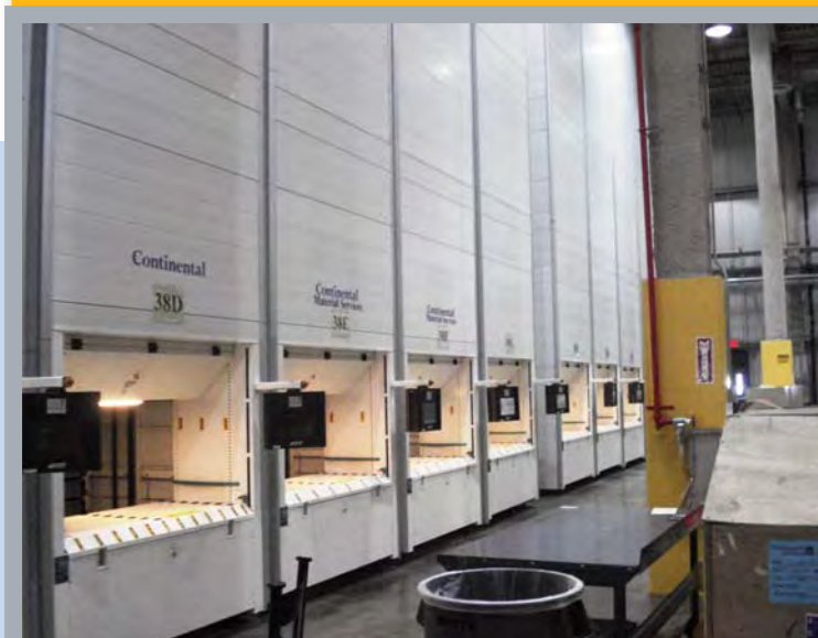
Savings in time, space and a cleaner, more secure parts inventory are among the benefits of using VLMs over static shelving.
